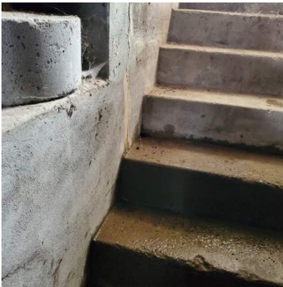
3.4.5.7 During the wettest months, groundwater seeps into the basement.
