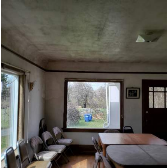
3.4.5.5. The interior is starting to show signs of moisture and mildew staining.
