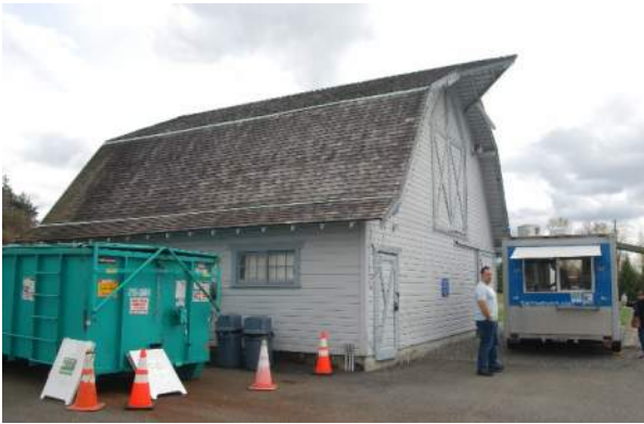
Photo 3.2.5.1: The front façade of the barn facing 104 th Street. Note the hay hood at the roof peak.
