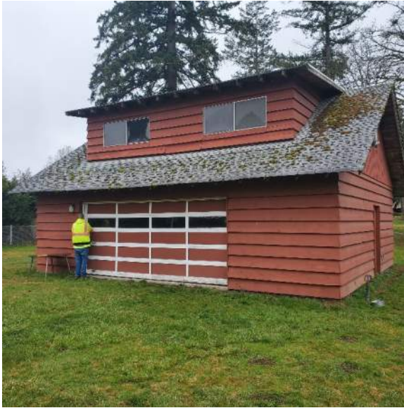
3.3.5.1 The front east elevation. The sectional garage doors are 7-foot high doors.
