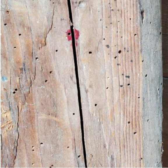
Photo 3.2.5.5: The tiny pin-sized holes are evidence of powder post beetles. Their primary food source is wood. They can damage a building's structure.
