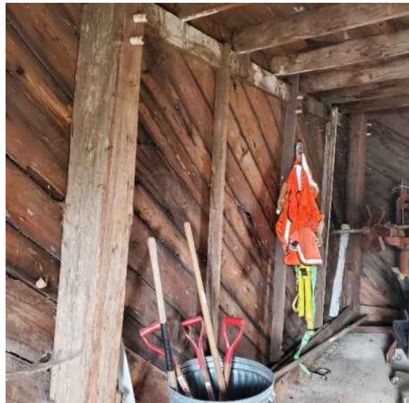
Photo: 3.1.5.4: The primary structure is timber poles and lumber. The sheathing is diagonal boards.
