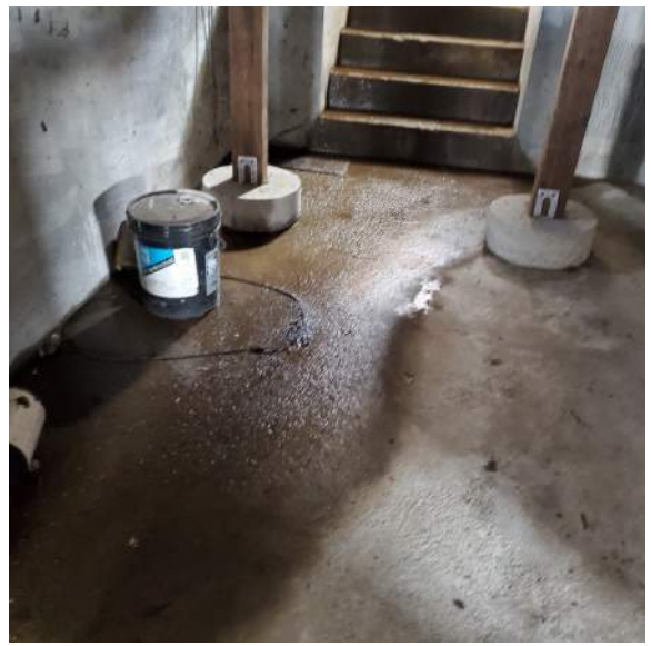
3.4.5.8 The first floor structure had to be repaired at some point. Note the new plinths underneath the posts.
