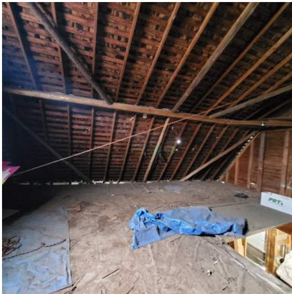
Photo 3.2.5.3: A view of the loft space and the barn's roof structure. Note the log poles for the primary structure and the sawn lumber for the roof joists.
