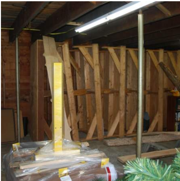
3.3.5.6. More storage of the Friends of the Park. Note the shoring under of the joists.
