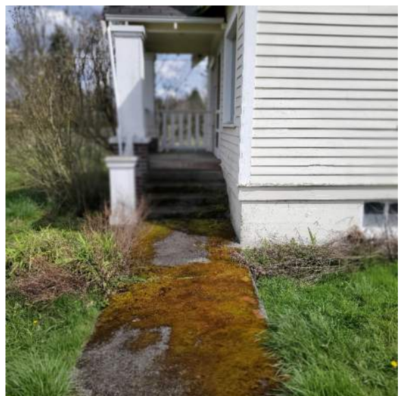
3.4.5.4 The walkway to front door would be a barrier to making the building accessible.
