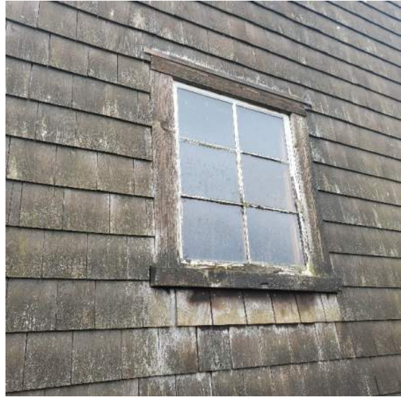
Photo 3.1.5.2: The exterior siding is wood shingles. Note the weathering of the window sash.
