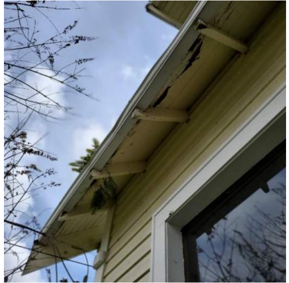
3.4.5.2 The eave at the northeast corner of the building is showing water damage. The gutter appears to be blocked and there are ferns growing in it.
